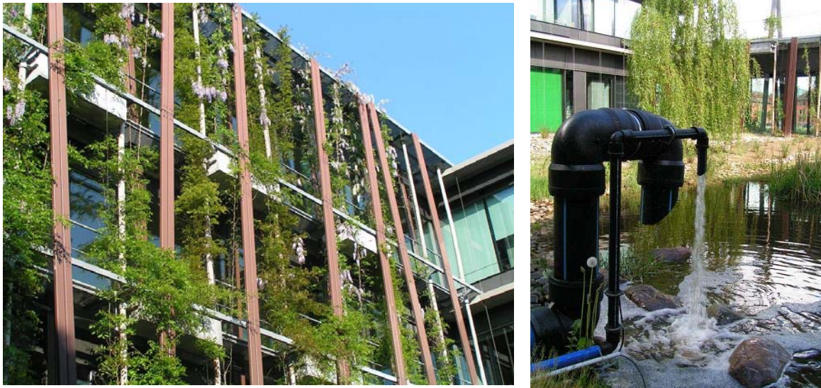
Figure 10: Façade greening system (priority 2).
