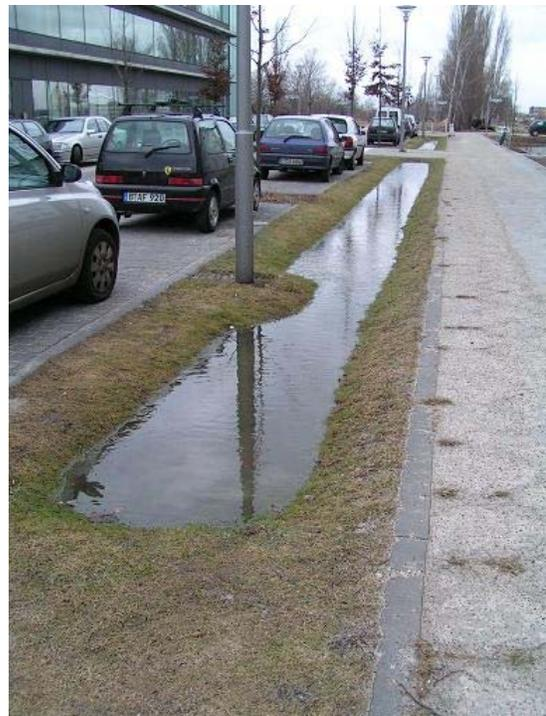
*Figure 6: Trough infiltration system in Berlin, lacking vegetation (priority 7)*
