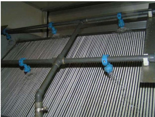
*Figure 12: Adiabatic exhaust air cooling with rainwater in seven air conditioning systems (priority 4)*
