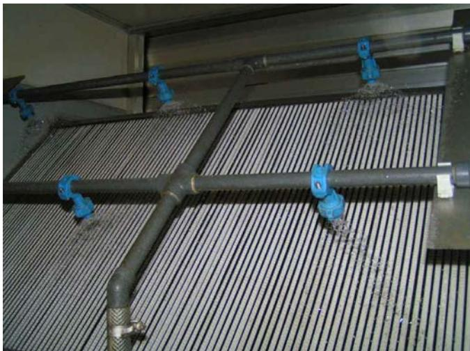
**Figure 2** adiabatic exhaust air cooling in seven air conditioning systems
