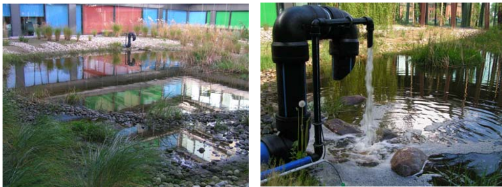
Figure 3, 4 constructed lake with natural surface infiltration inside of a courtyard
