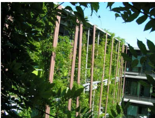
Figure 4 façade greening system, Institute of Physics, Berlin-Adlershof
