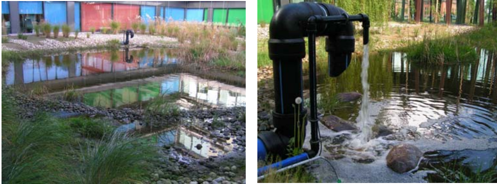
Figure 2, 3 constructed lake with natural surface infiltration inside of a courtyard
