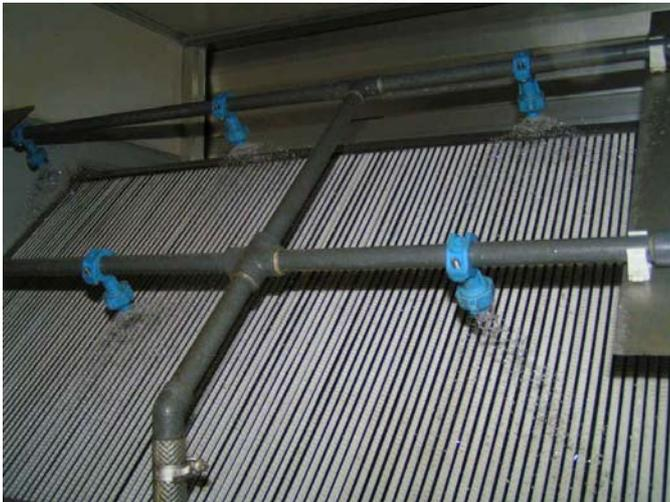
**Figure 5**      adiabatic exhaust air cooling in seven air conditioning systems
