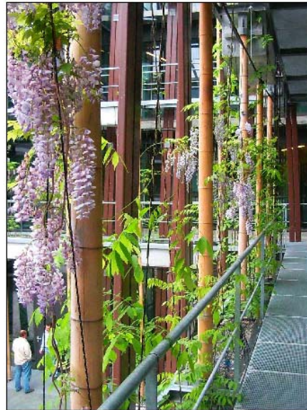
Figure 1 façade greening system, Institute of Physics, Berlin
