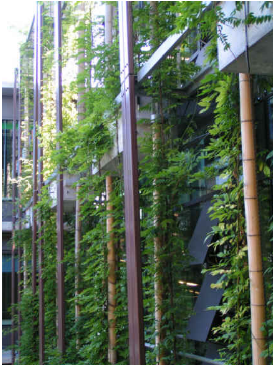
Photo 3 Climbing plants at the institute of Physics in Berlin provide shade and cooling by evapotranspiration
